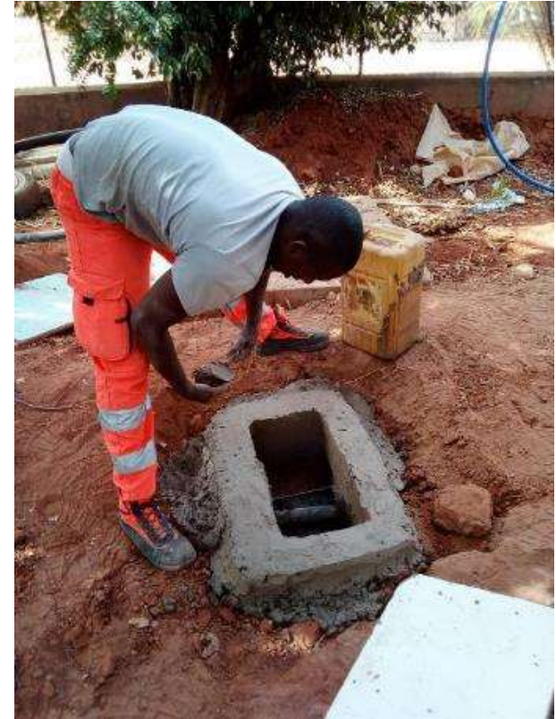
Sewer inspection construction
