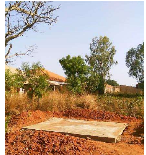
Stand foundation for drinking water tank...
