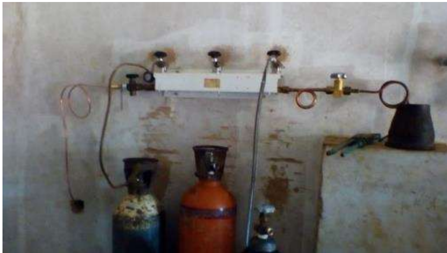
Both boosters are simultaneously operating to fill the cylinders with medical oxygen (94-96% purity)
